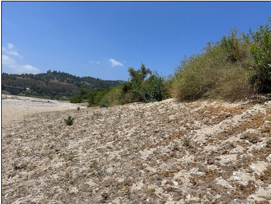
Photo 10: Overview Side Slopes
