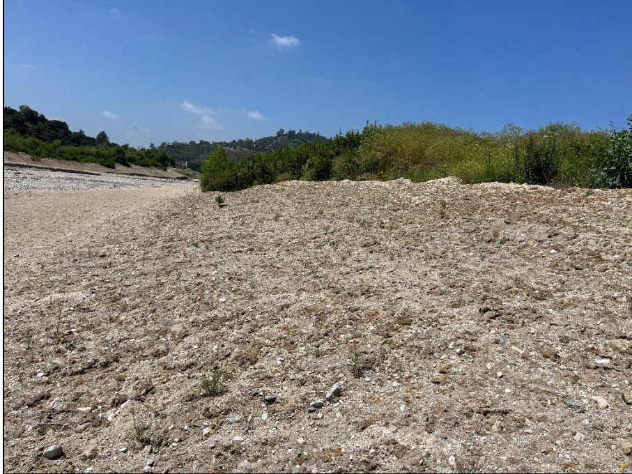
Photo 11: Overview Side Slopes
